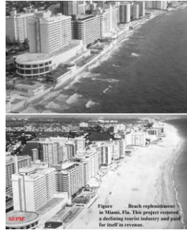
Figure Beach renourishment in Miami, Fla. This project reversed a declining tourist industry and paid for itself in revenue.
